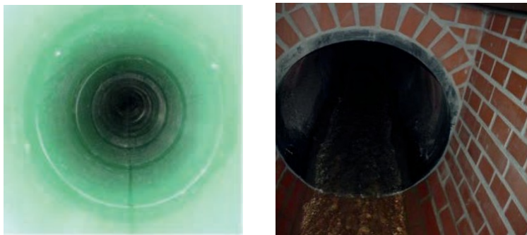
Figure 6: Left: Pipe rehabilitated using the tight-in-pipe method. Right: Manhole connection
