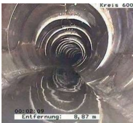
Figure 4: Rehabilitation with the tight-in-pipe method (left: before rehabilitation, right: after rehabilitation)
